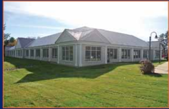
5 Industrial Parkway, Brunswick
